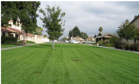
Turf block fire access road, Santa Clara
