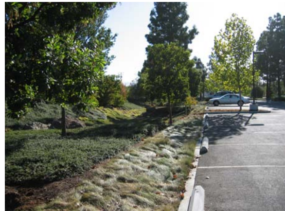
Parking lot runoff drains to a detention basin in Palo Alto.
